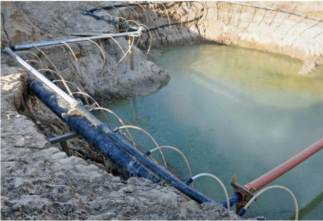
Ground water dewatering
